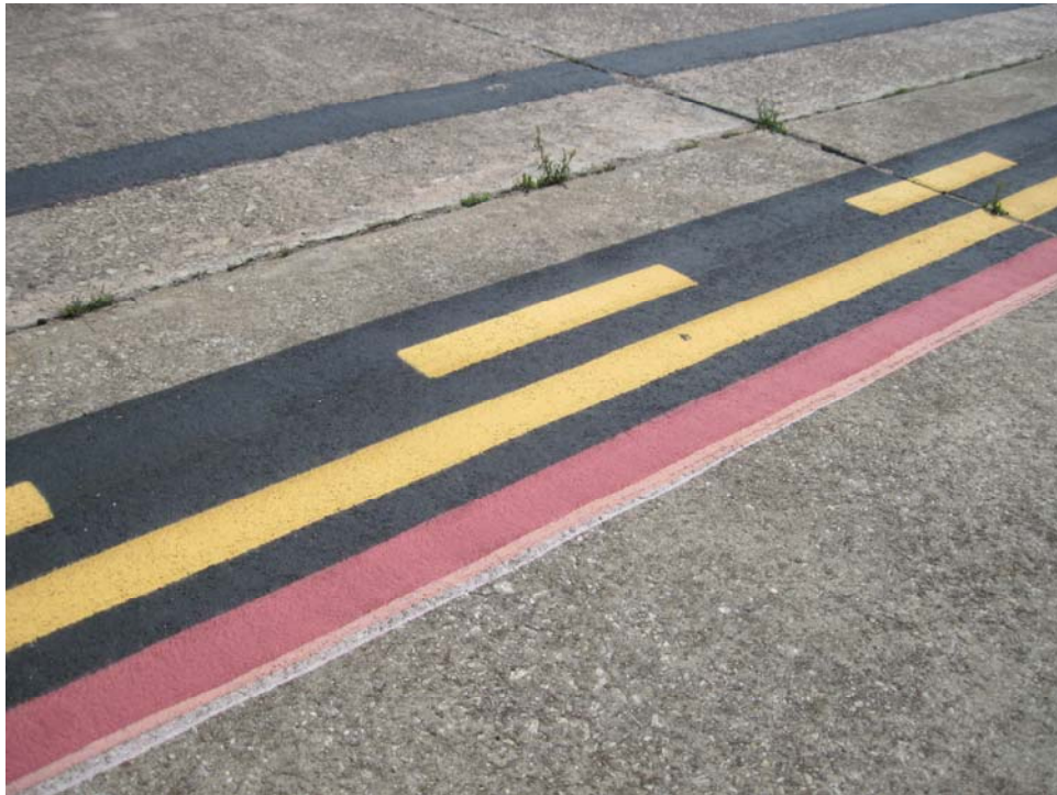
ANWRAMPAP-20. Satisfactory Paint.
