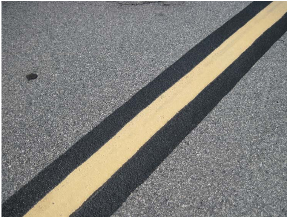
ANWRAMPAP-10. Satisfactory Paint.
