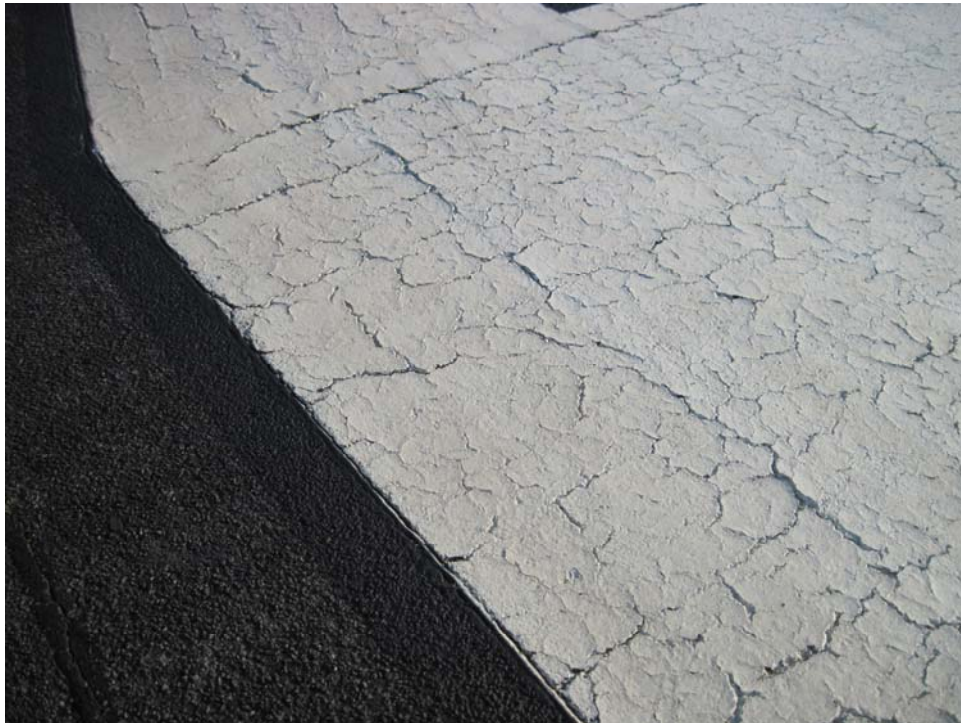
R1634AP-10. Satisfactory Paint.
