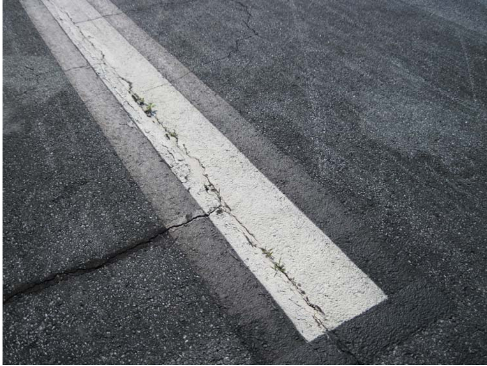
R927AP-10. Satisfactory Paint.
