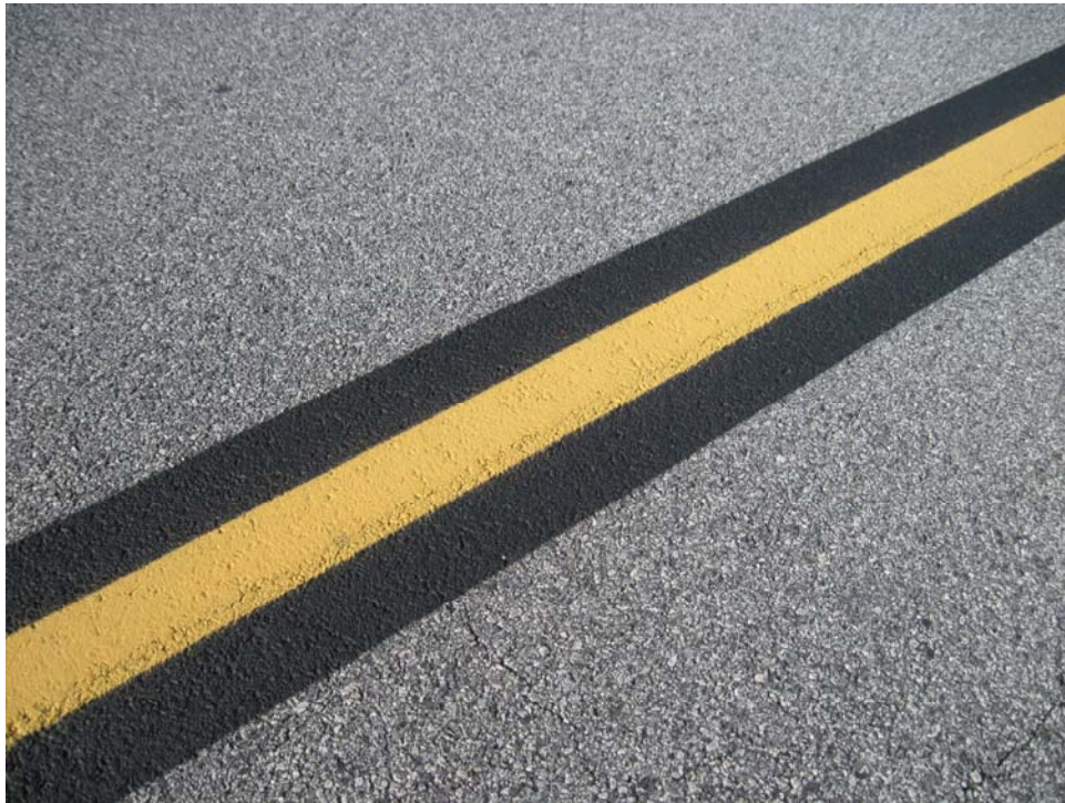
TCAP-20. Satisfactory Paint.
