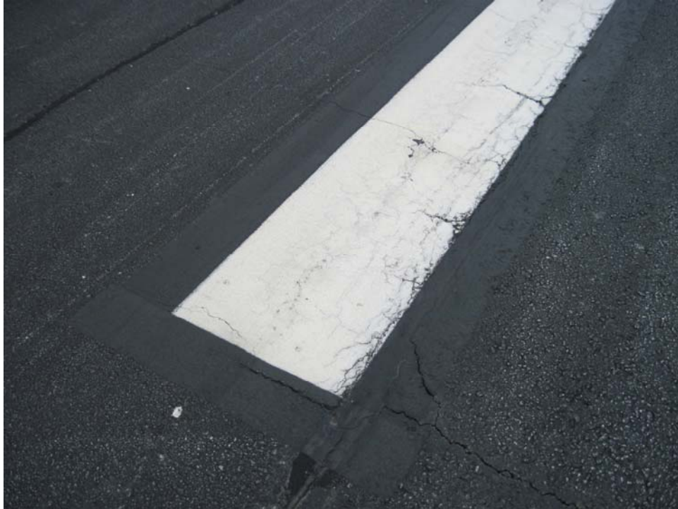
R2L20RAP-10. Satisfactory Paint.
