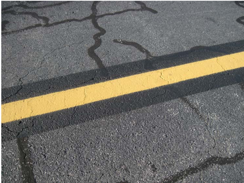
TCAP-30. Satisfactory Paint.
