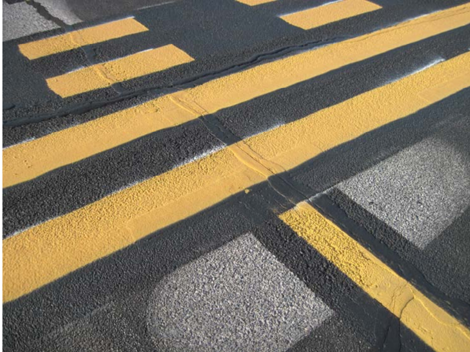
TBAP-40. Satisfactory Paint.
