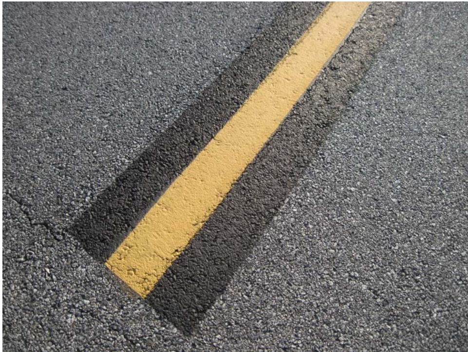
TBAP-30. Satisfactory Paint.
