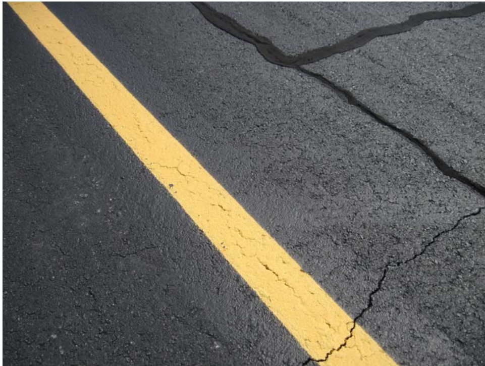
TDAP-10. Satisfactory Paint.
