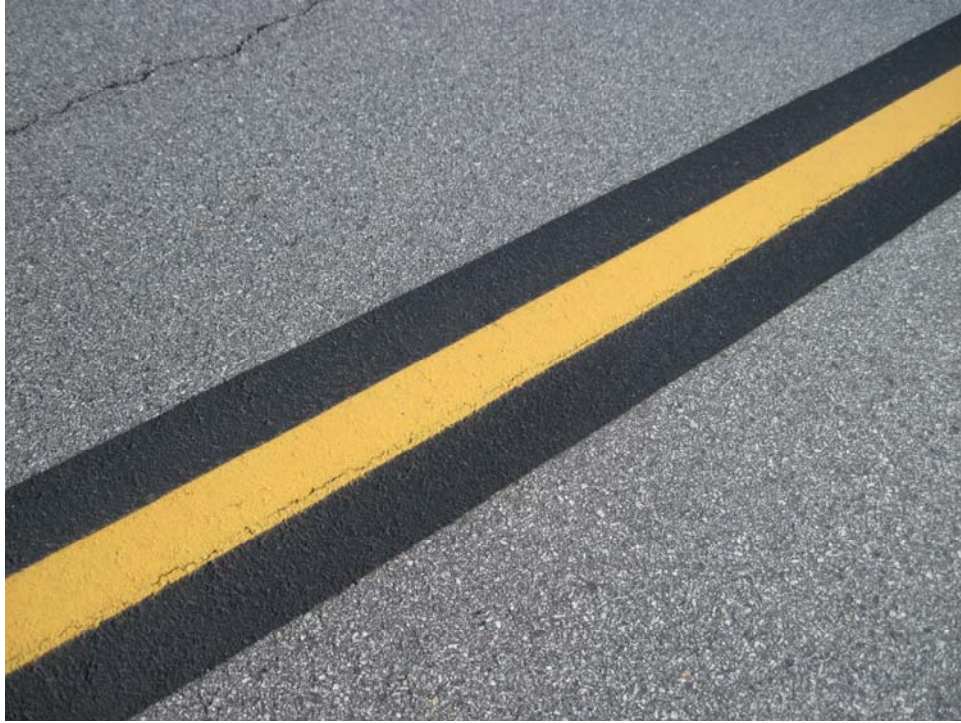
TCAP-10. Satisfactory Paint.
