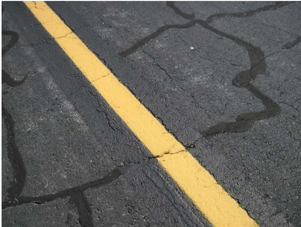
TBAP-10. Satisfactory Paint.
