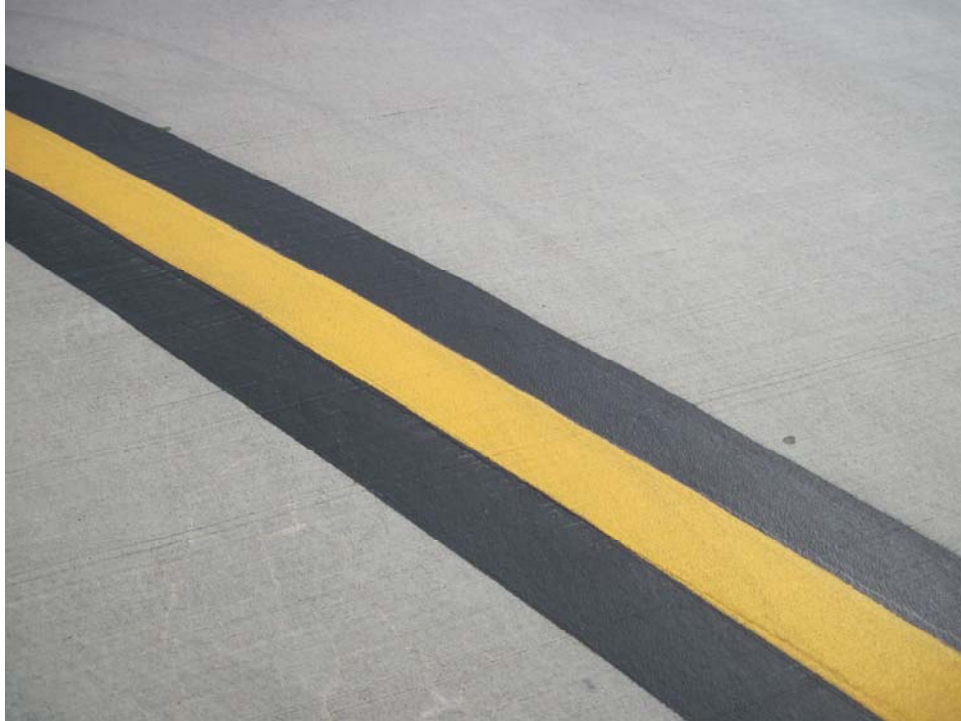
TARUNUPAP-10. Satisfactory Paint.
