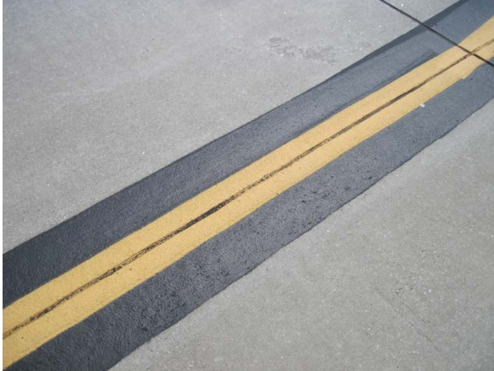
TBAP-20. Satisfactory Paint.
