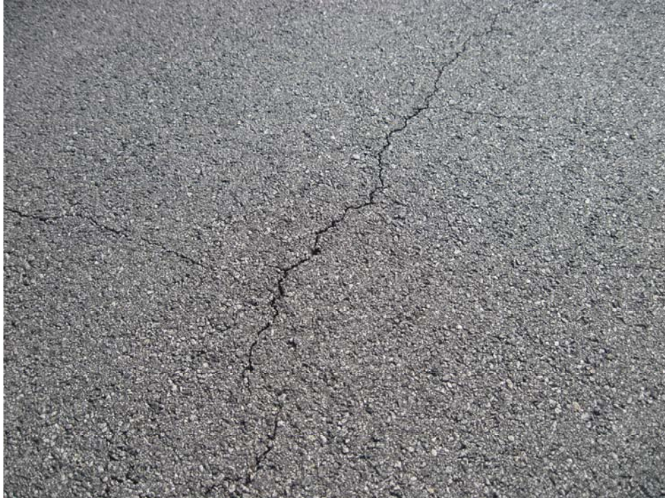
TCAP-20. Weathering and Longitudinal and Transverse Cracking (Sample Unit #01).
