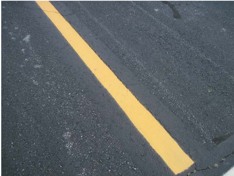
TGAP-10. Satisfactory Paint.
