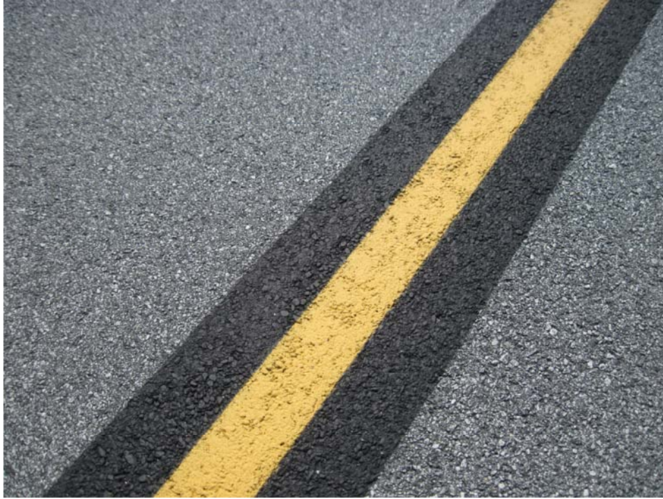
TDAP-20. Satisfactory Paint.
