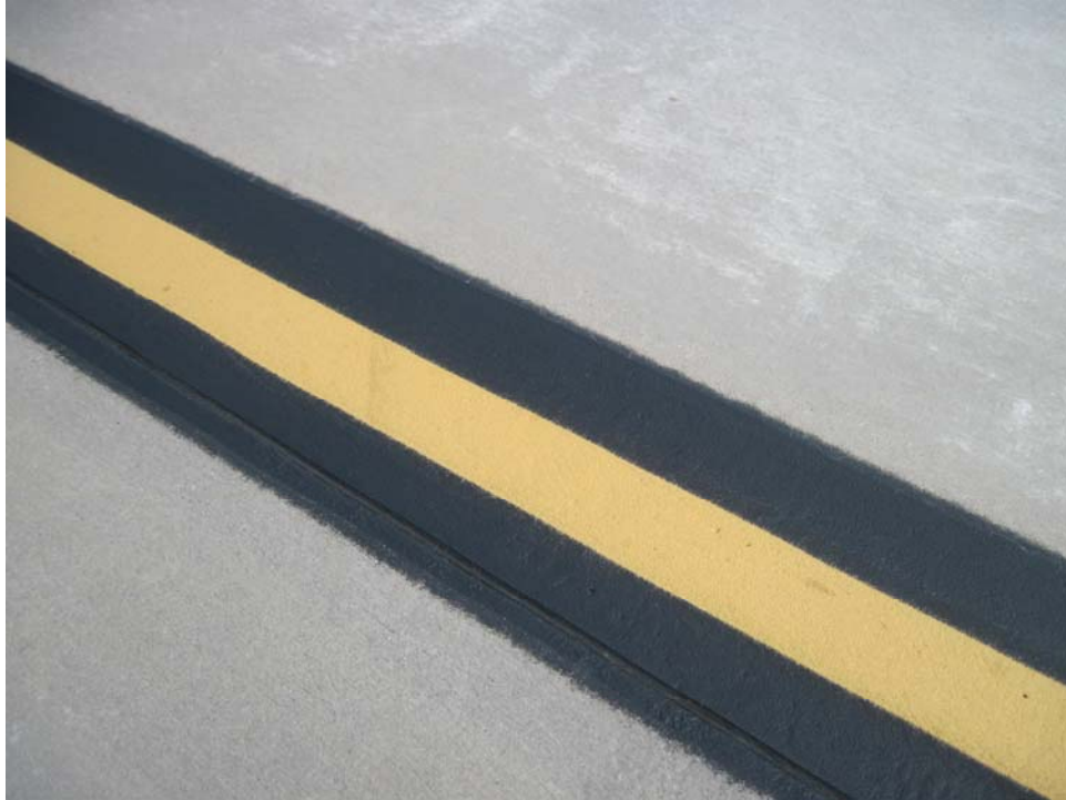
THAP-10. Satisfactory Paint.
