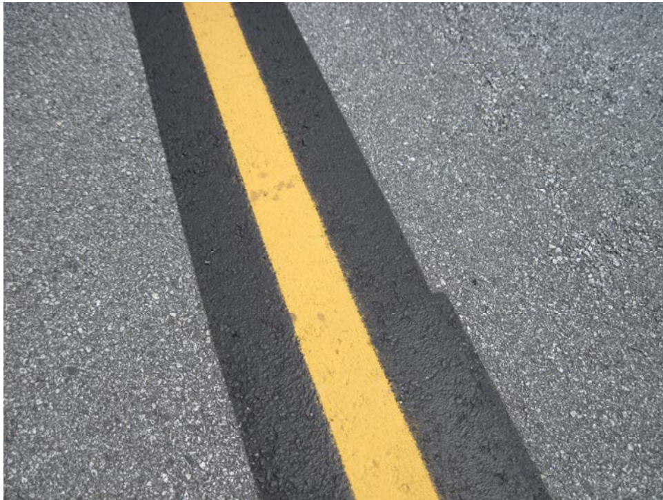
TFAP-10. Satisfactory Paint (1).
