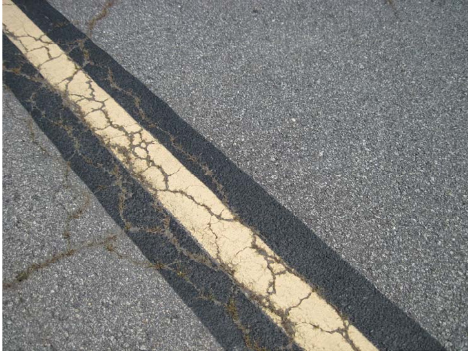
ANRAMPAP-10. Satisfactory Paint.
