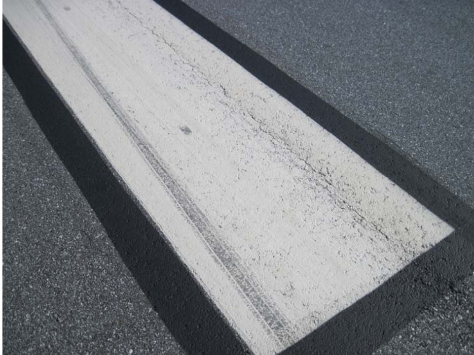
R1634AP-20. Satisfactory Paint.
