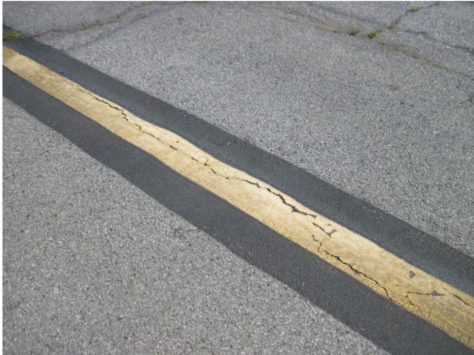
ANERAMPAP-10. Satisfactory Paint.
