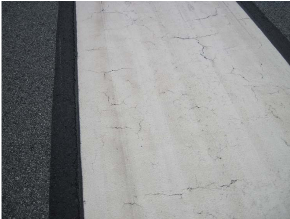
R2L20RAP-20. Satisfactory Paint.
