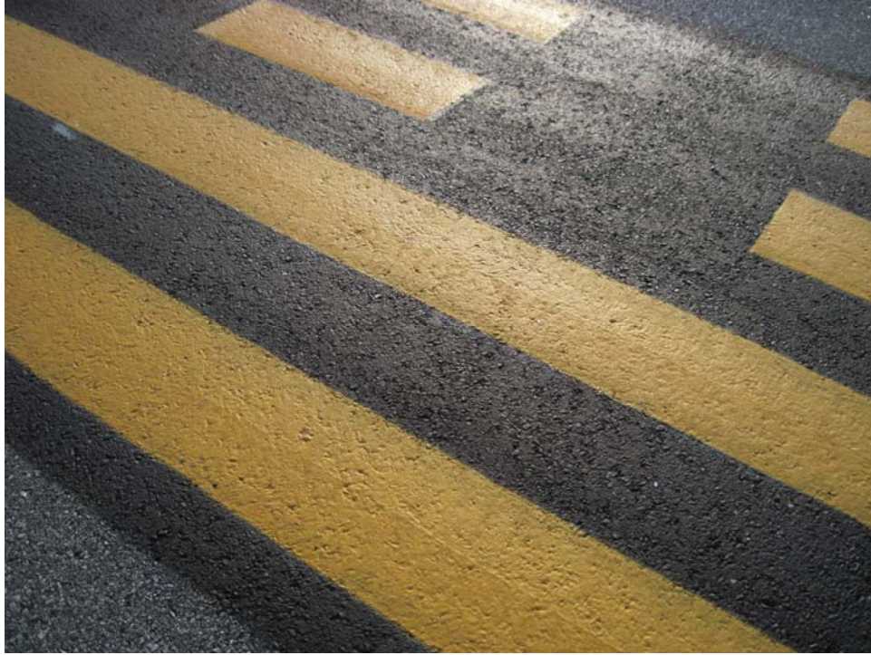
TFAP-10. Satisfactory Paint (2).
